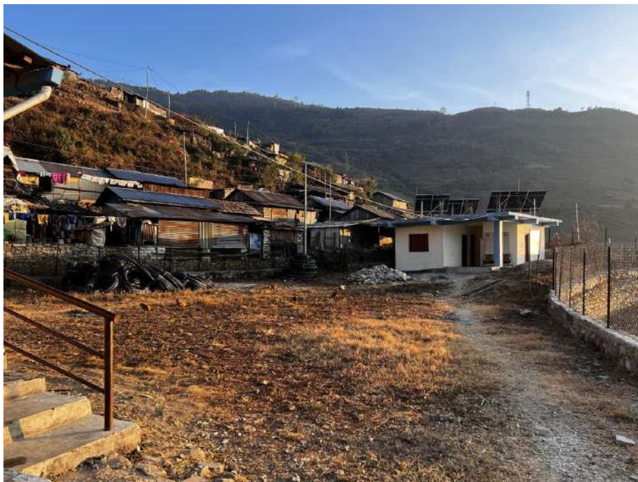
The site where the new building will be constructed
